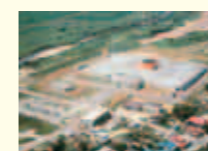
Takahata (Yamagata) Plant completed (1974)
